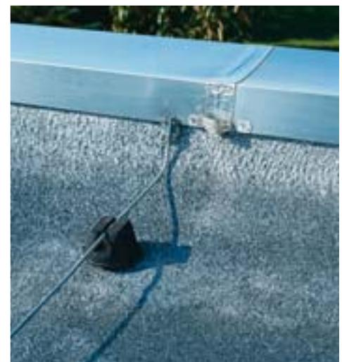
△△△ Critical points such as parapets, domelights or, as shown here, ventilators, are sealed without difficulty using Elastopor H.
