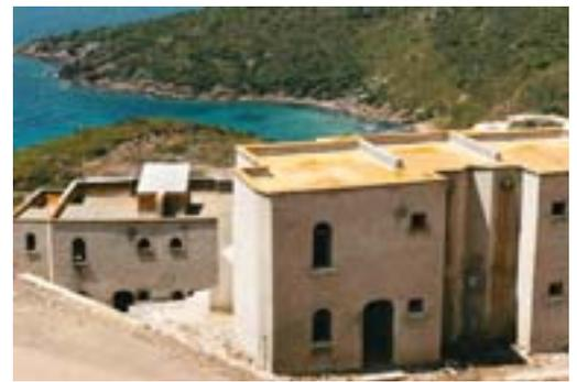
*△ Altogether 12,000 m<sup>2</sup> flat roofs with allround parapets and coated with Elastopor H. Holiday apartments in Bodrum, Southern Turkey. In southern climates, the thermal properties of Elastopor H ensure an agreeably cool room temperature.*
