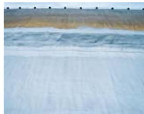
△△ The old fibre production in Premnitz, near Berlin, was renovated one roof after another. The economic solution for insulating and weatherproofing: Elastopor H. The roof in the foreground is already completely coated with Elastopor H and already partly covered with a protective coating against UV light.
