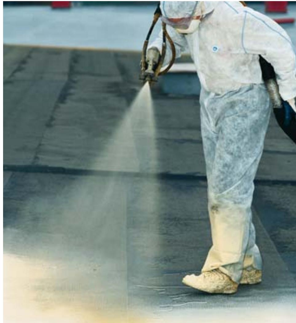
Experience shows that roof sealing with Elastopor H spray foam systems gives savings in time of up to 80% and savings in cost of up to 50% as compared with conventional methods. An experienced processing team can cover more than 1,000 m<sup>2</sup> of roof surface per day with one machine under favourable conditions.
