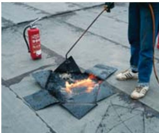
*△ Preparation stage: after cleaning the roof one can spray over the old bitumenised roofing felt. Large blisters or loose areas must be glued down to provide a firm substrate.*
