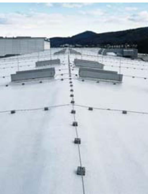
*△ 4,900 m<sup>2</sup> corrugated sheet and flat roof of a paint factory in Oberhausen coated with Elastopor H.*
