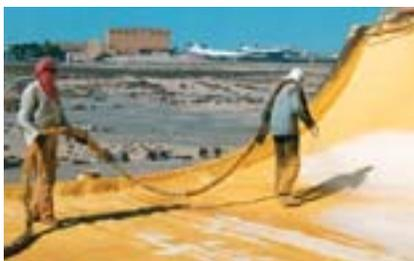
*△ 44,000 m<sup>2</sup> of roofing of the airport building at Abu Dhabi, United Arab Emirates, coated with Elastopor H and protected with a UV resistant paint.*
