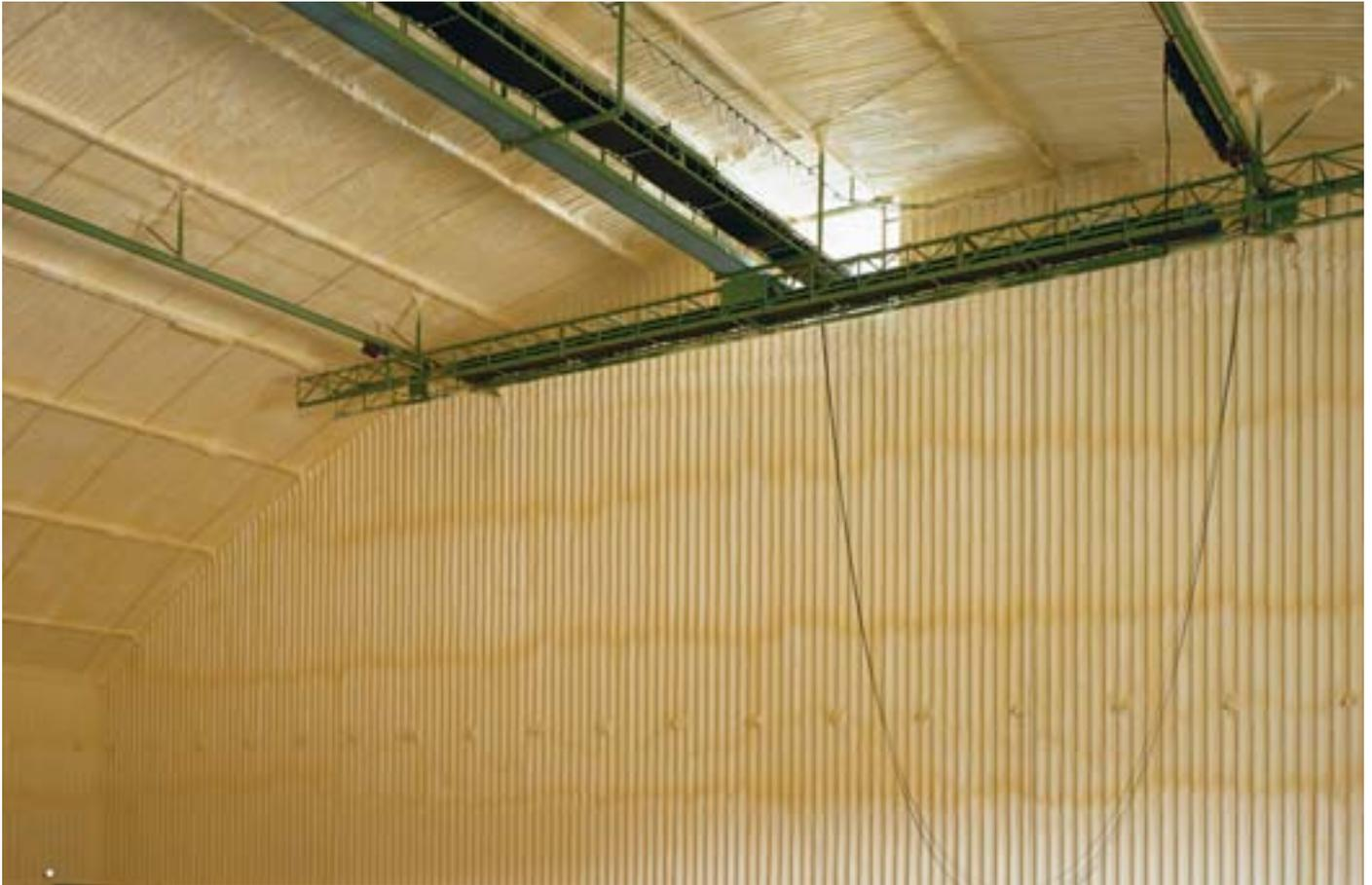
*△▷ This 16,000 m<sup>2</sup> grain store in Essen, Oldenburg, with an external steel skeleton construction is thermally insulated from the inside and made airtight: with Elastopor H.*
